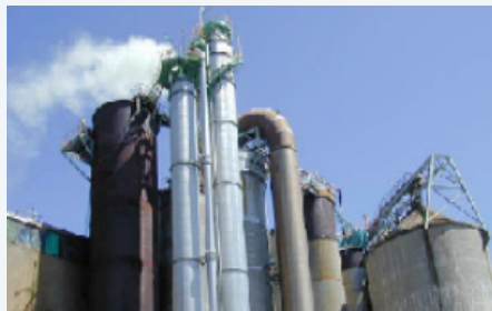
BLEACH PLANT & NEW O2 DELIGNIFICATION TOWERS
