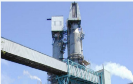
KAMYR CONTINUOUS DIGESTERS
